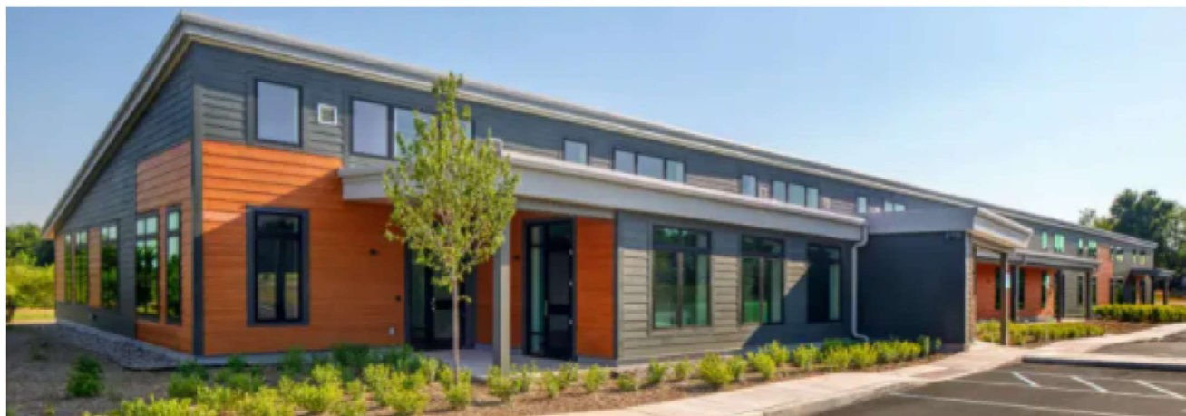
Sustainable Energy Fund (SEF) office building Schnecksville, Pennsylvania.
