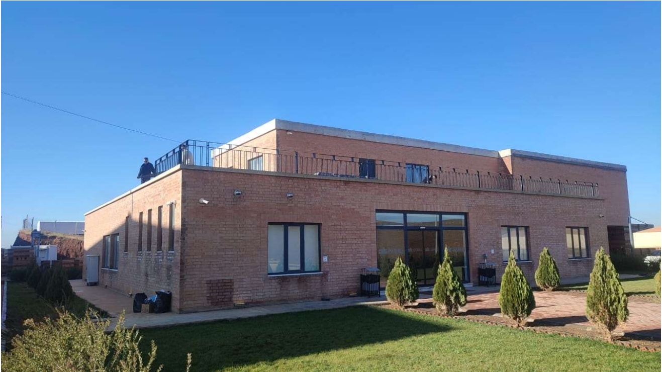
Administration Building of Ashur Brick Company in Chamchamal district External and Internal walls built by Iraqi standard Brick (Common Brick 24x11.5x7.5cm), Hollow block slab with bricks used in construction of Slabs
