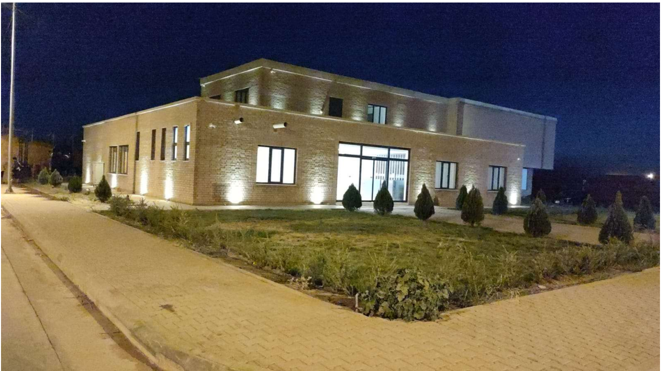
Administration Building of Ashur Brick Company in Chamchamal district External and Internal walls built by Iraqi standard Brick (Common Brick 24x11.5x7.5cm), Hollow block slab with bricks used in construction of Slabs
