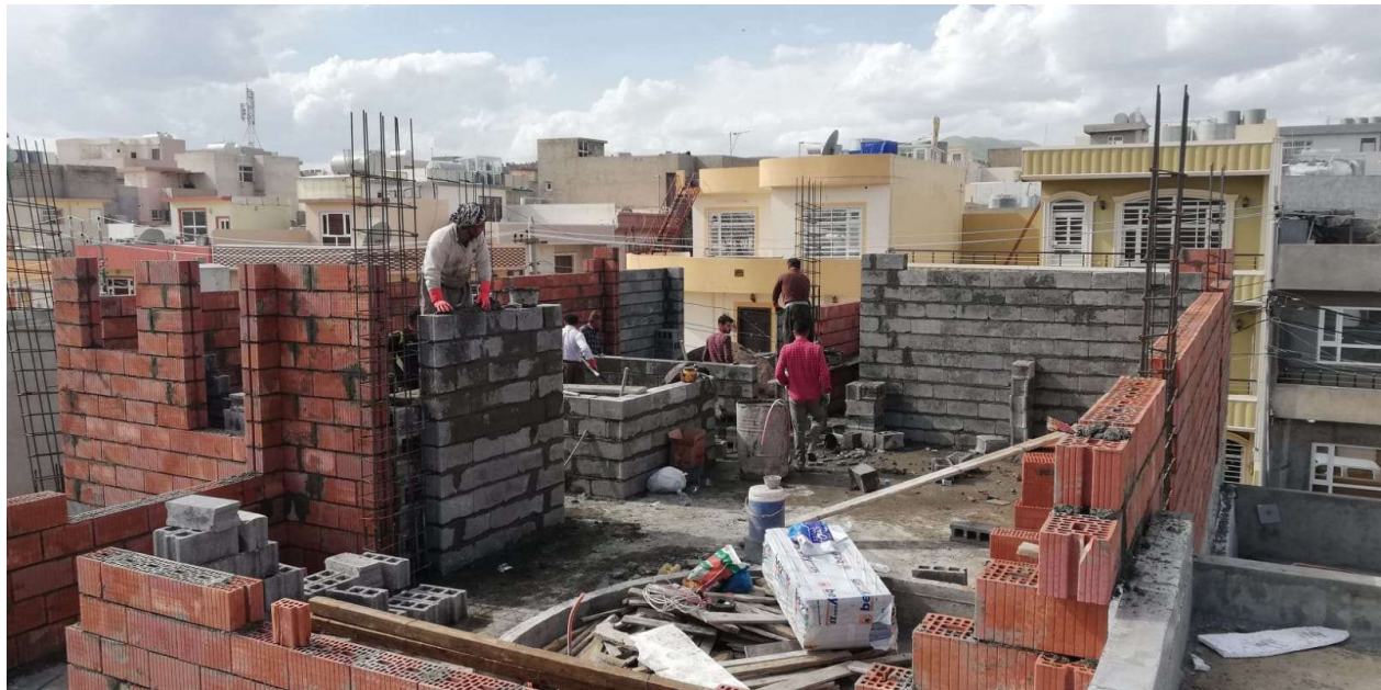
Construction of New Building ( Practical Case Study )
